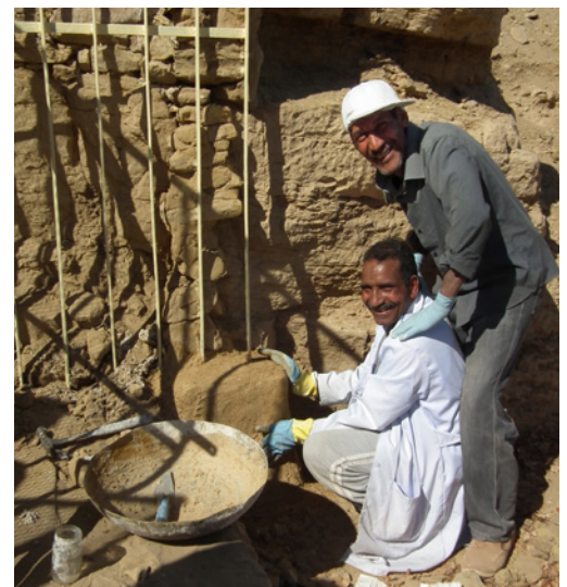
Prince and Abdel Setar reinforcing the gates for extra security.
