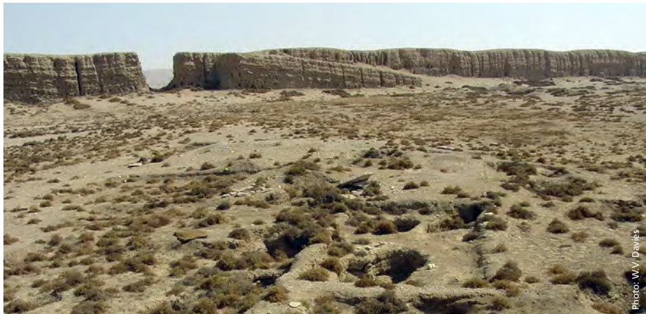
The massive Late period walls of Elkab rising over 10m in height surround the remains of earlier settlements still buried deeply below.
